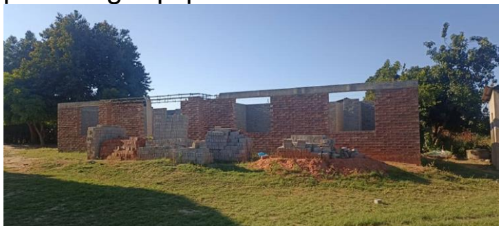
Rectory under construction
