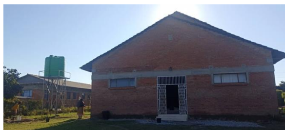
Church building and the water tank
